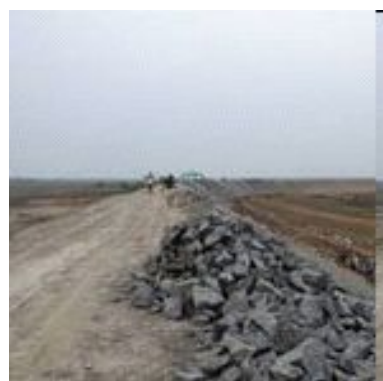
Rajnagar, Gopalpur Saline Embankment Balasore District, Odisha
