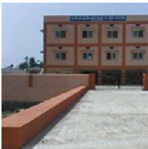
Cyclone Shelter at Palmanpeta, Visakhapatnam District, Andhra Pradesh
