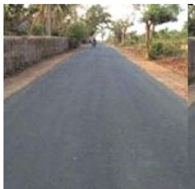
Bitumen (BT) Road in Matikhola, Ganjam District, Odisha
