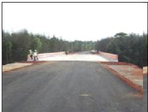
Puligedda Bridge, Vijayanagaram Dist, Andhra Pradesh
