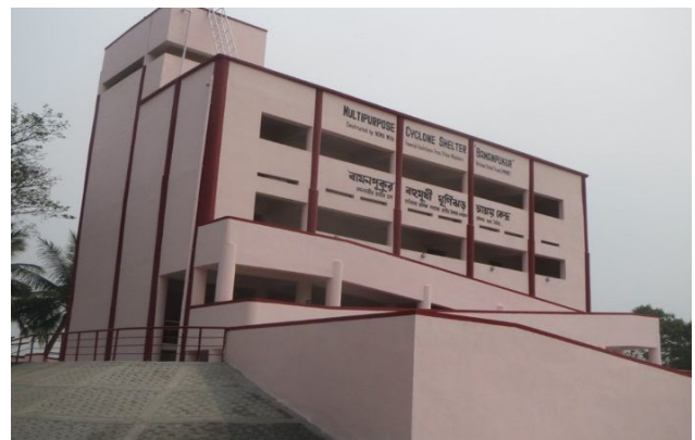
Cyclone Shelters at Kaushangra, North 24 Parganas District under PMNRF
