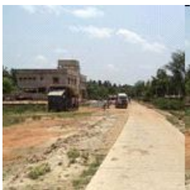
Cement Concrete (CC) Road, Panchubisa, Odisha
